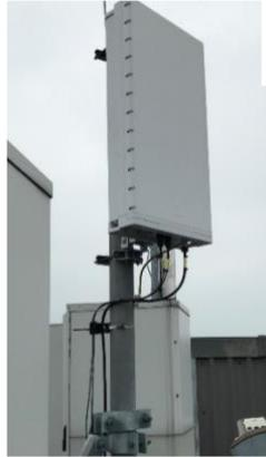
Figure 16: 5G NR AAS for use in the 3.5 GHz band
